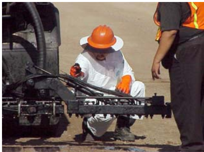
MCDOT Employee Examines Equipment Before Operating to Assure Quality
