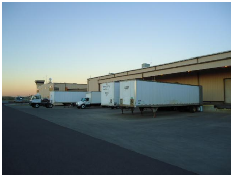
Boeing's Distribution Center in Mesa Arizona
